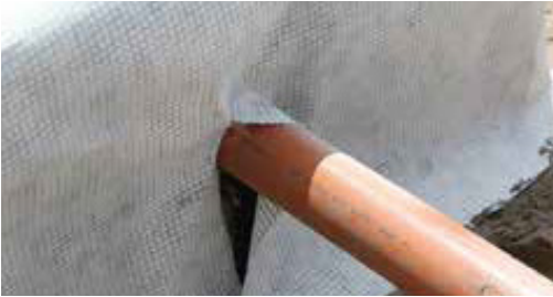
Make a straight cut in the TP combigrd around the TreeParker system up to the height of the utility.
