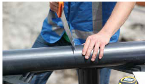
The TP posts can be cut with a hand tool or machine on top of the system.
