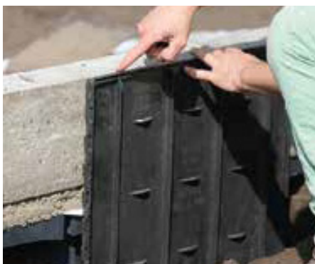
The bottom should be at least 5cm deeper as the soil surface inside the system.
