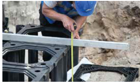
Measure the needed height.
