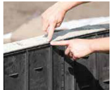
The top of the panels should be above the soil surface around the tree.
